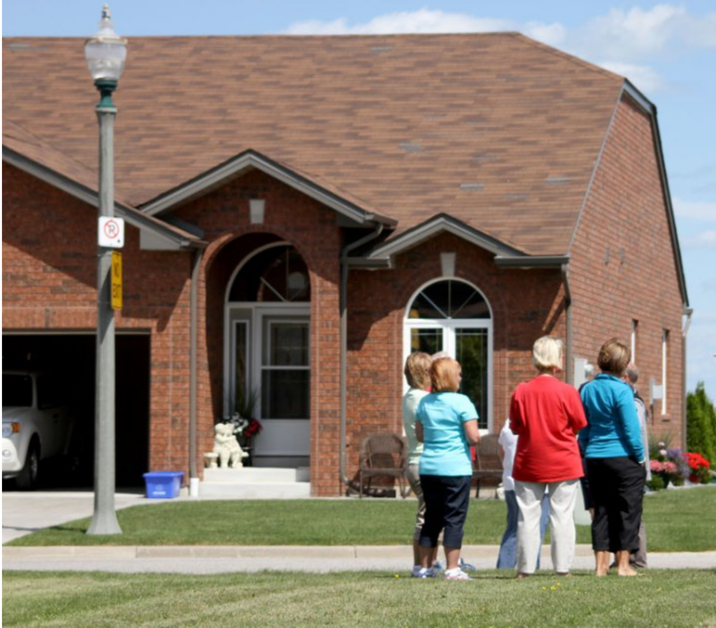
Homeowners on Aspen Shore Avenue stand outside a home with some missing shingles. (RICK DAWES / The Windsor Star)
